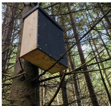
Figure 27 The box in its final position and with all the installation equipment removed
